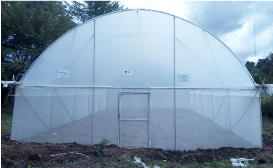
Green house installed at Cheptengis Okilgei Women Group in Cherangany ecosystem
